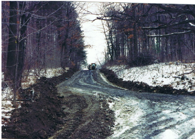
Bishop Road, February 26, 2009. Temperatures at or near freezing result in our snow plows doing damage to dirt roads that lack sufficient gravel cover, when trying to plow slush off the roads.
