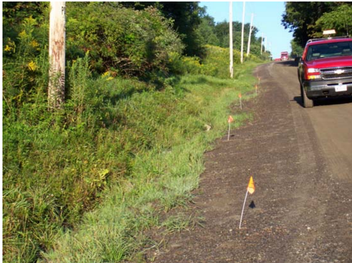
Bishop Road prior to starting work on it, September 2009
