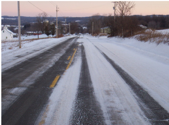
One of the more problematic drifting areas on Stagecoach Road December 21, 2008. Fifteen minutes after this was taken a deep snow drift had crossed over the road again.
