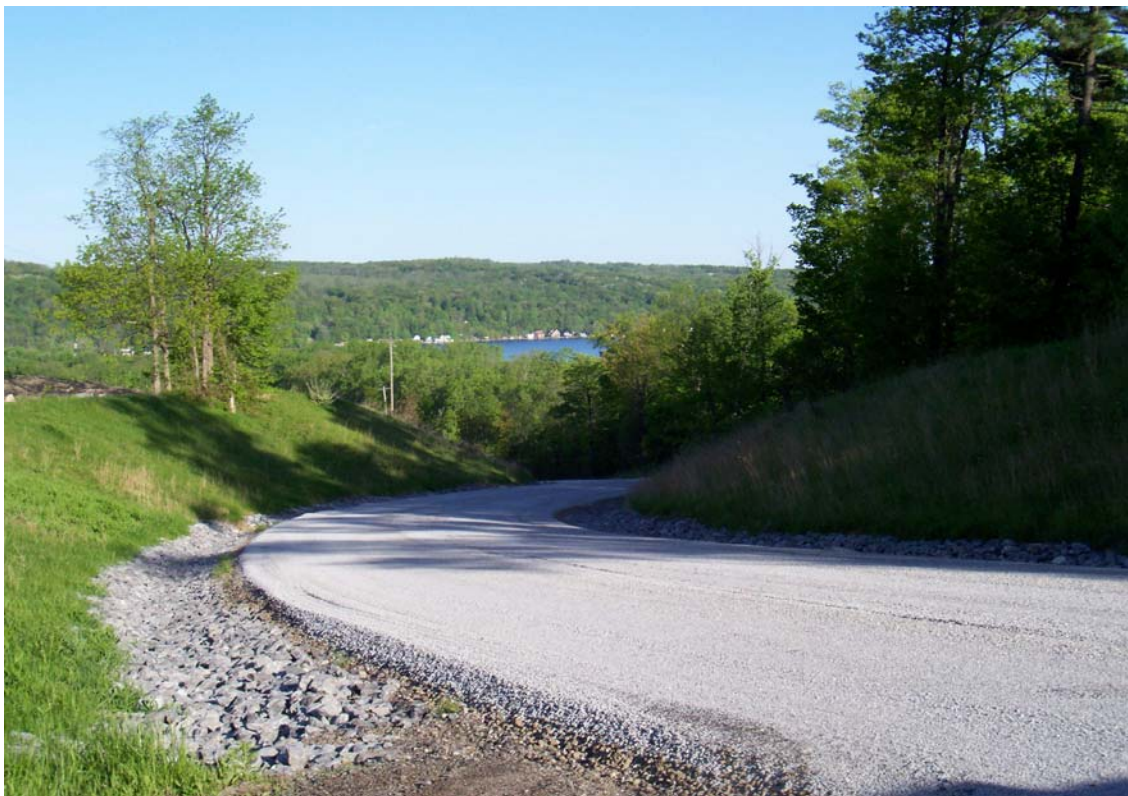
Taken after the road was oil and stoned on May 14, 2009. With the roadbed sealed the danger of road bed eroding is completely negated.
