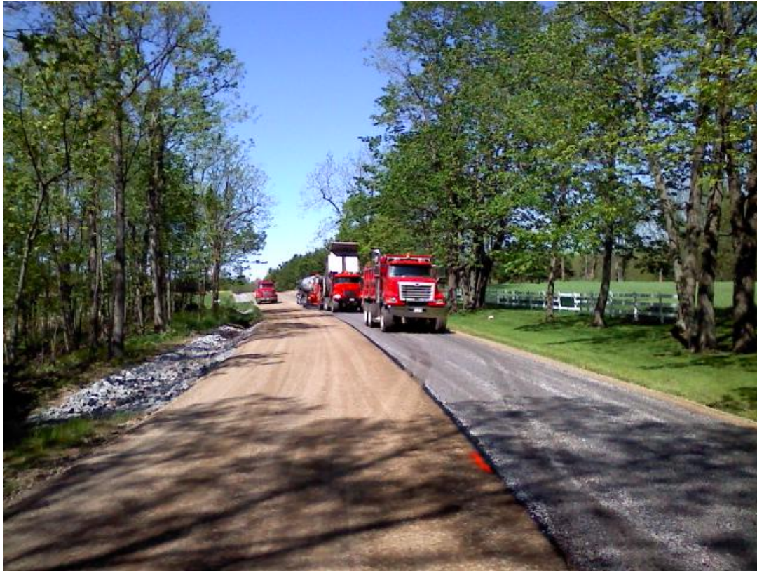
Oil and stone being applied to Henderson Hill Road, May 2009
