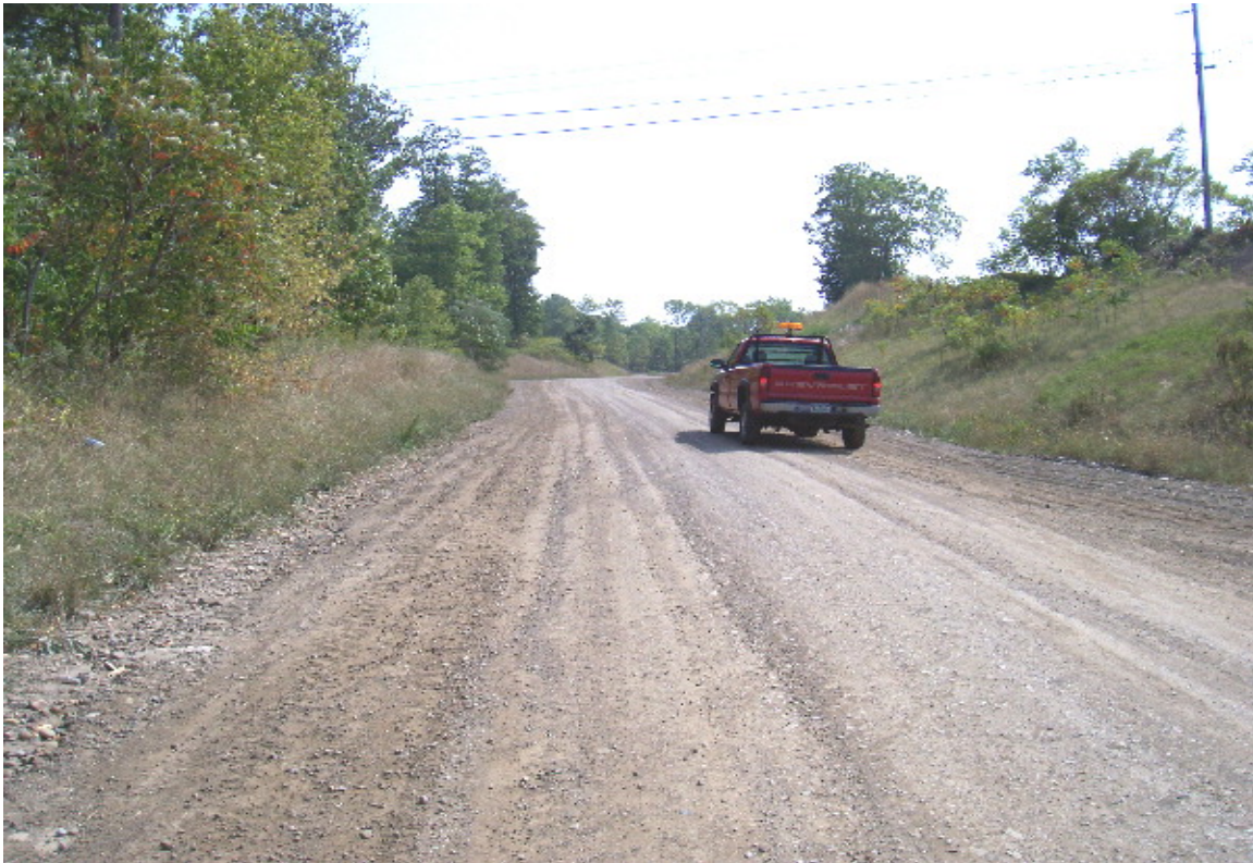
Henderson Hill Road on May 27, 2006. (Looking east)
